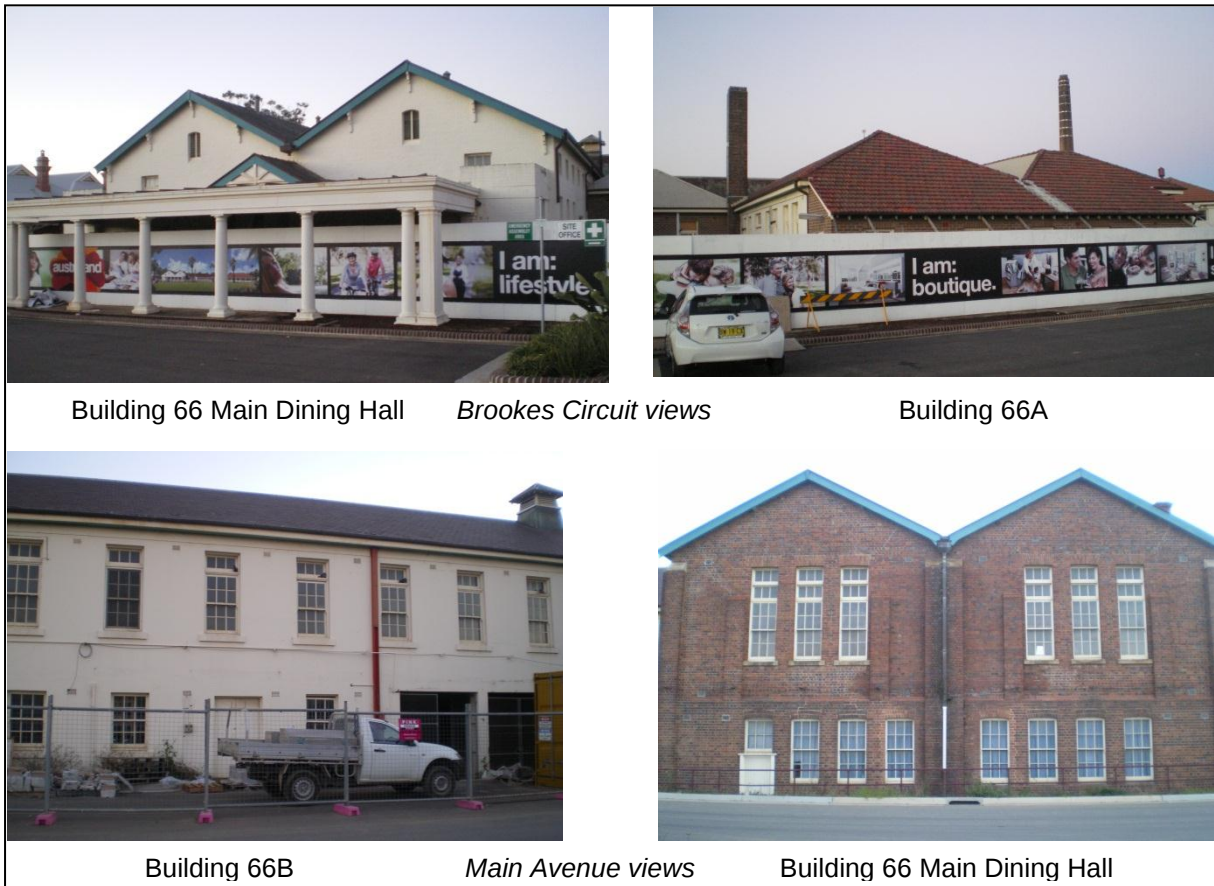
Figure 3: Views of Building 66
