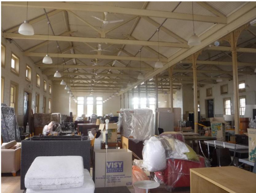
Figure 3 Interior of the former Dining Hall (Building 66), March 2011 (Source: GML, 2011)
